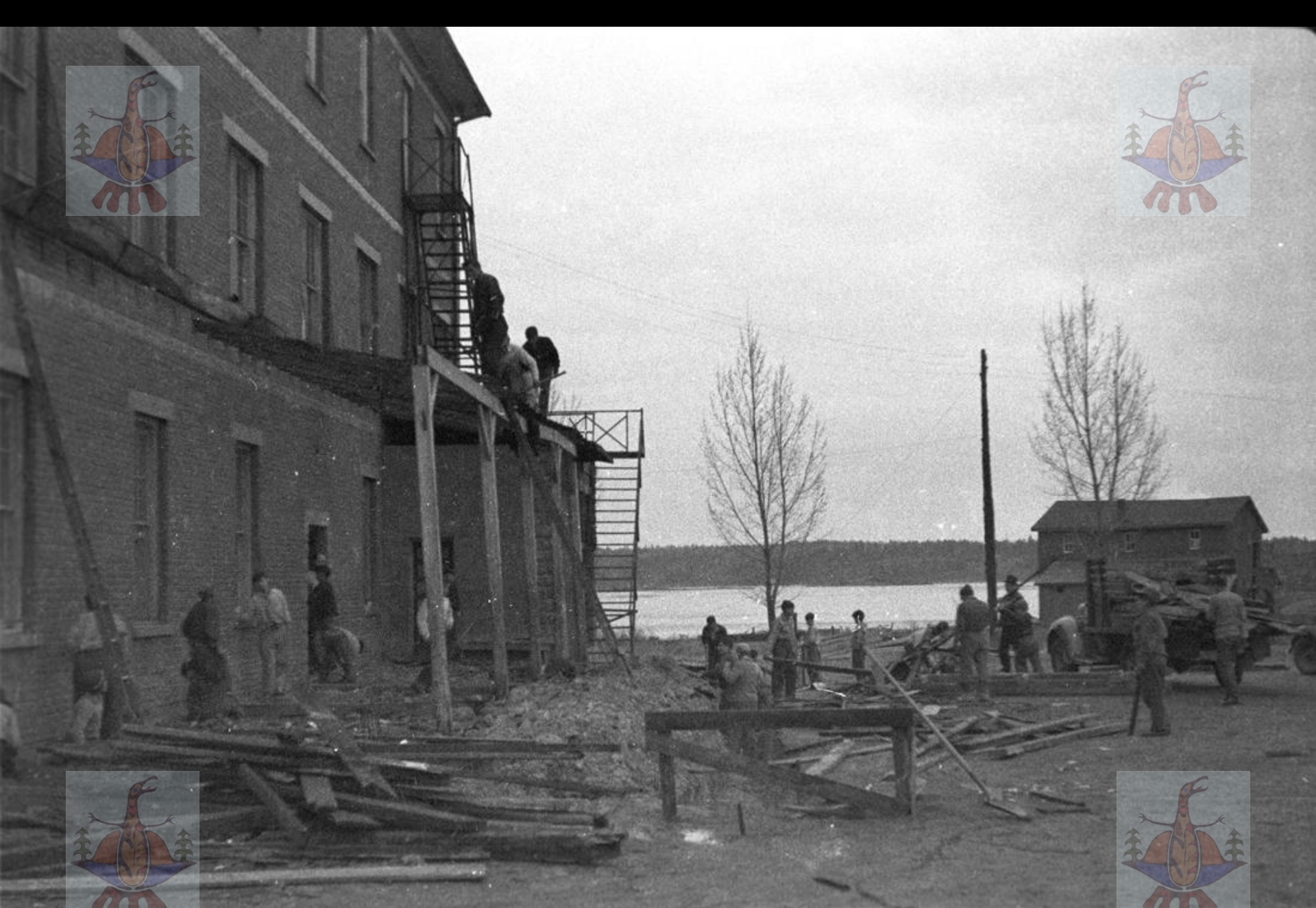
Old back verandah torn down (1952-1953)
