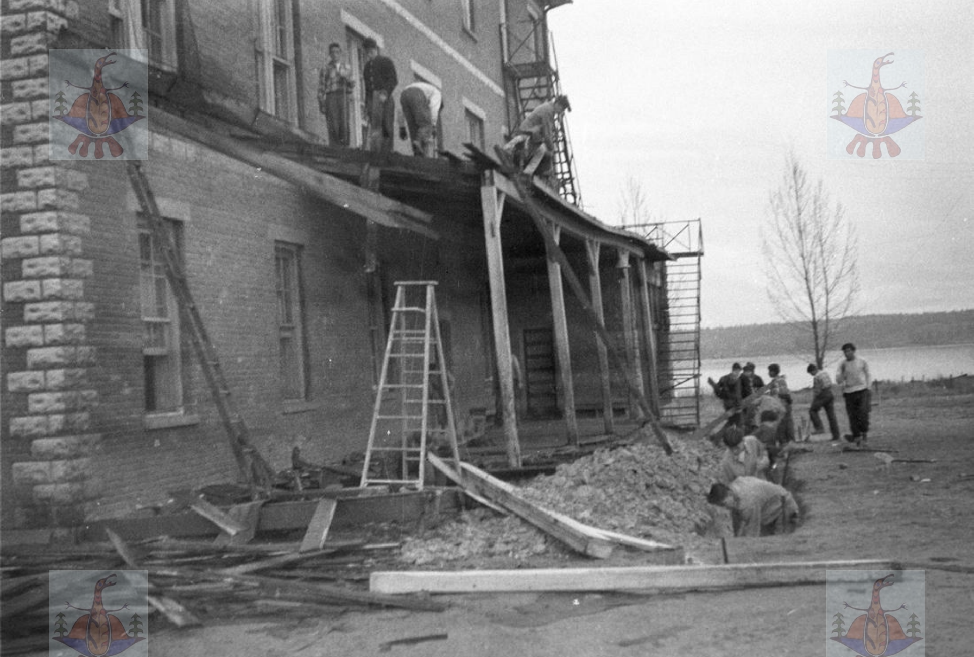
Old back verandah torn down (1952-1953)
