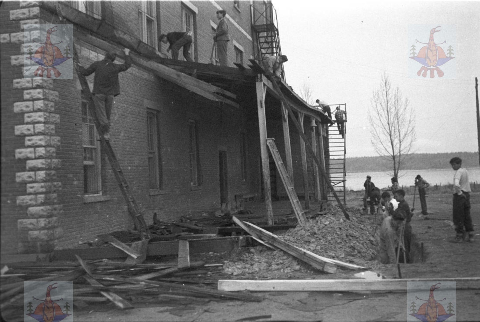
Old back verandah torn down (1952-1953)
