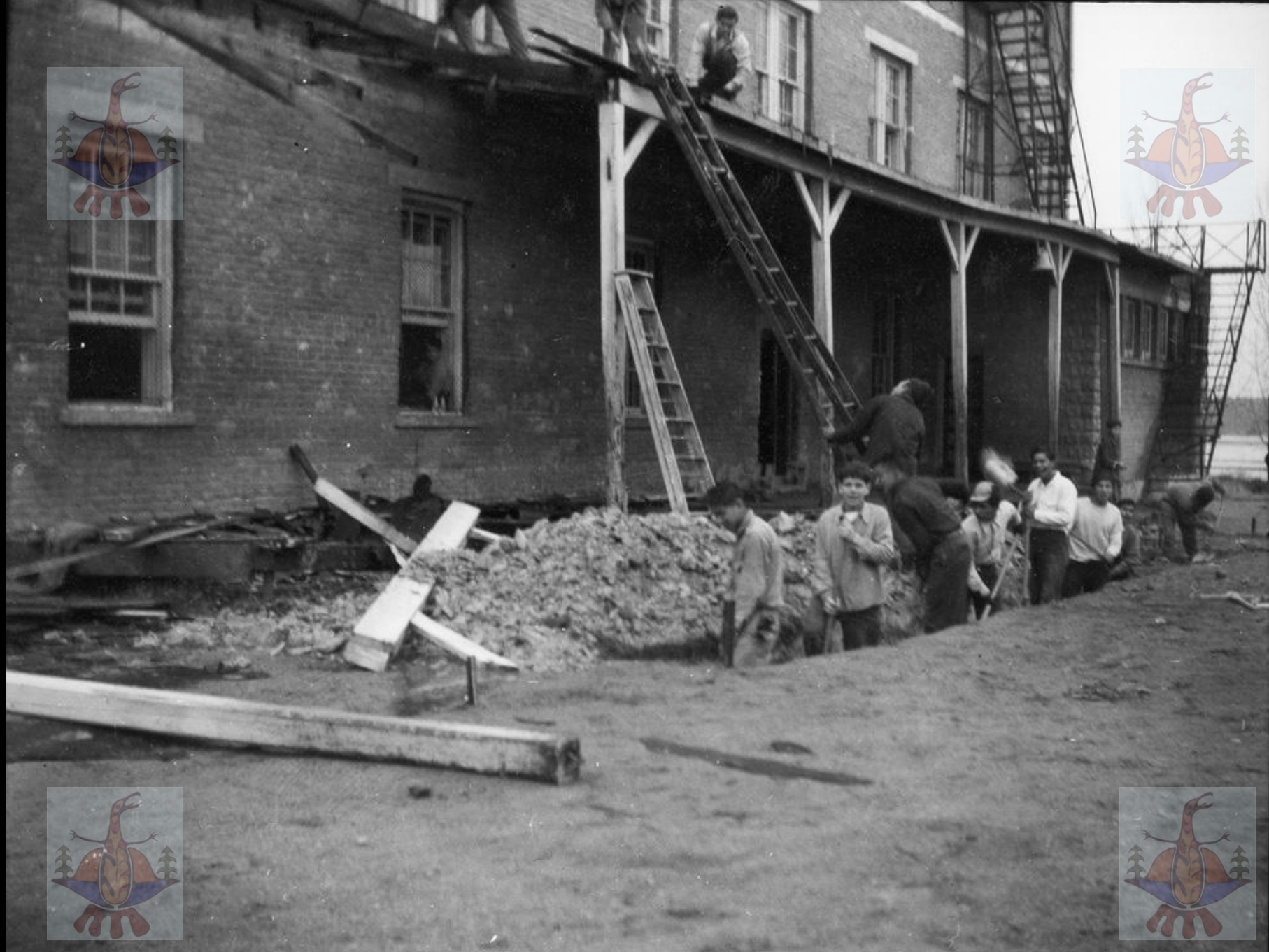
Old back verandah torn down (1952-1953)
