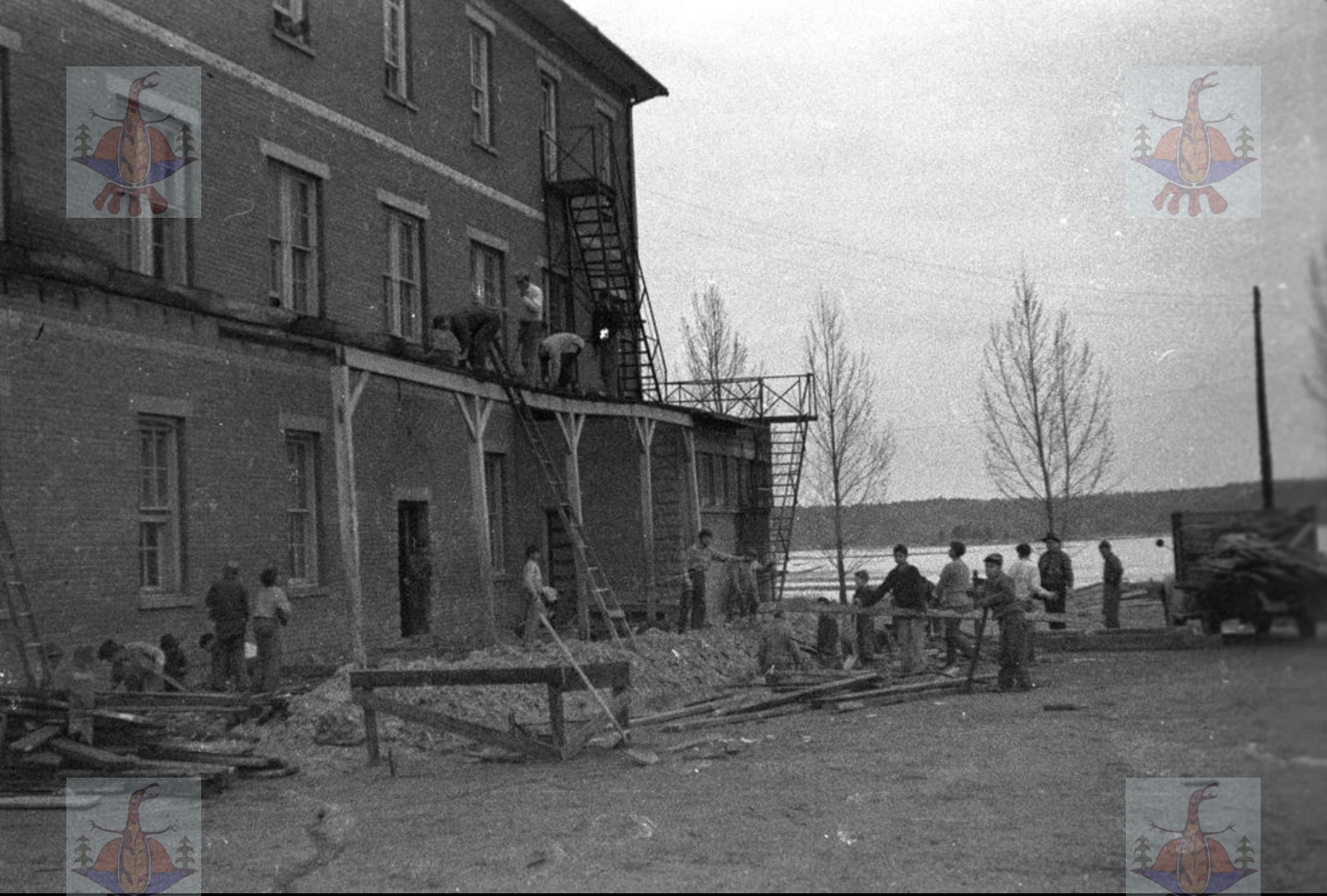
Old back verandah torn down (1952-1953)
